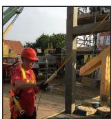
**8.** The driver will untie the blue rope then separate the 1st truss at the heel by hand or use of crowbar then replace the rope around the remaining trusses, repeating this process at the other end of the truss ensuring that, at all times, there is at least one rope securing the remaining trusses in the pack back to the centre bars.
