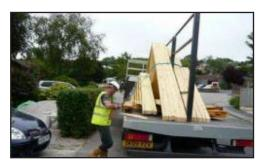
**4.** The manufacturer will supply truss packs secured to the trailer at two positions with 8 mm rope. Banded in packs (max 10 x 35mm/6x47mm) with yellow banding. You should familiarise yourself with which blue rope attaches which pack to the centre bars. Check each pack is roped separately.
