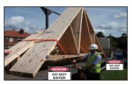
**6.** Ensuring the blue rope is holding the outer pack the driver will cut the yellow banding to allow separation of the individual trusses.
