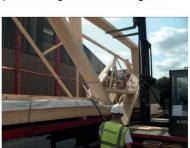
8. The forklift will then remove the truss pack from the trailer, position the apex of the pack onto the floor and reverse back slowly lowering the boom. Bearers can be used to support the underside of the pack.
